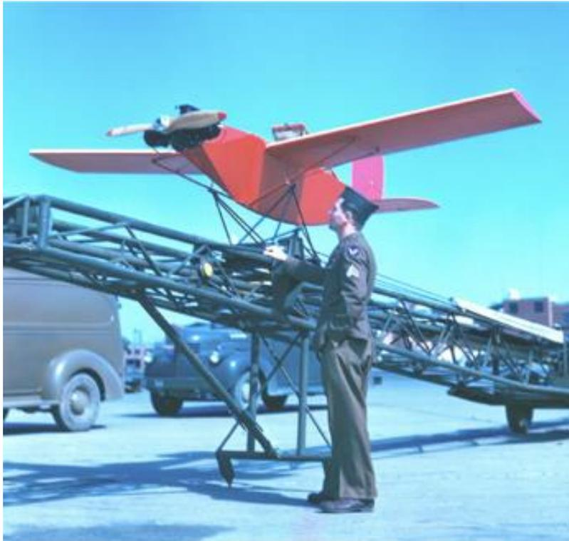
Figure 2 Radioplane OQ-3 on launch platform (wikimedia.org)
